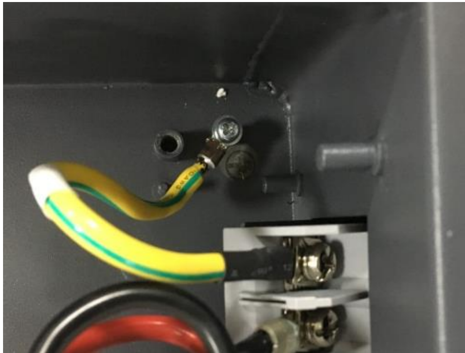
Figure 14 Earthing terminal
